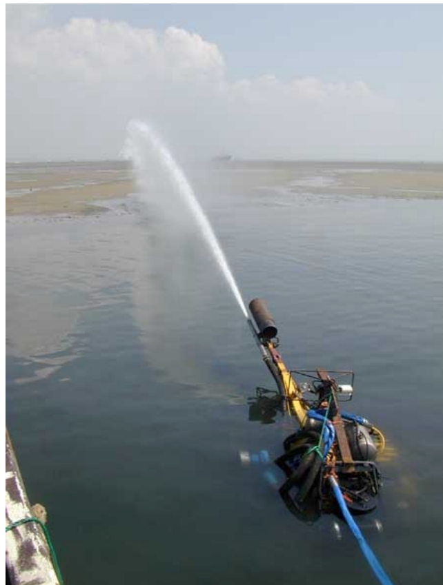
Testing the SBD2 jetting nozzles
